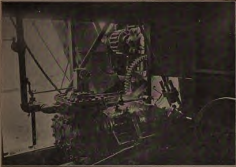
Spud Engine of Floating Dipper Dredge. Figure 82.
